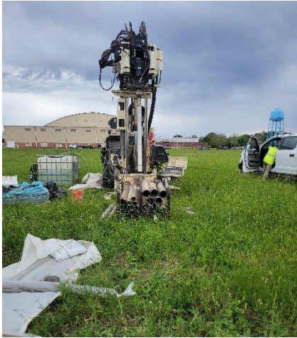
Figure 1: Monitoring Well Installation
